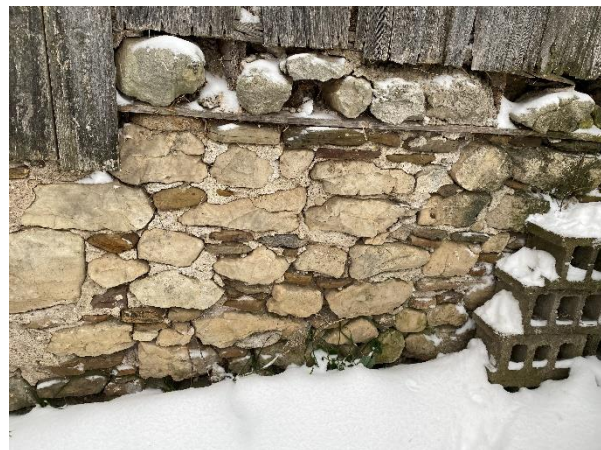
Plate 52: Detail of Barn No. 1 fieldstone foundations.
