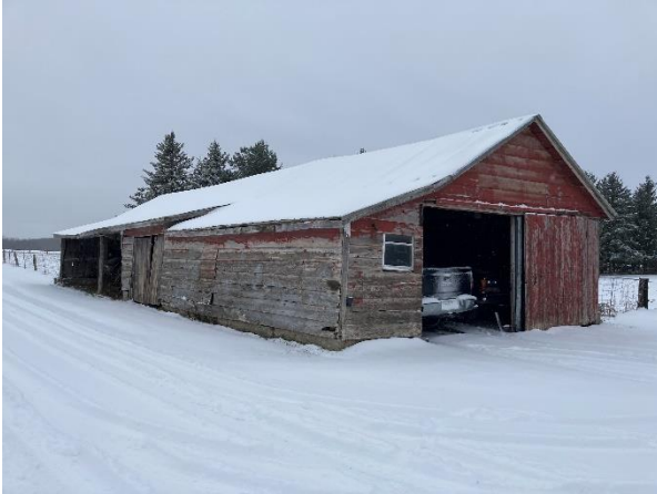
Plate 59: North and east elevation of Outbuilding No. 1.
