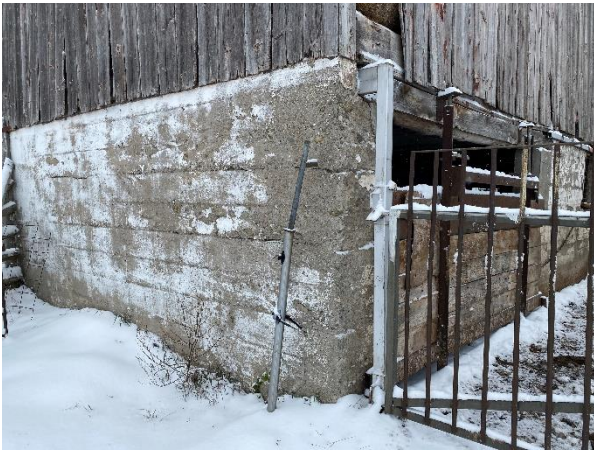
Plate 55: Concrete foundation of Barn No. 2.
