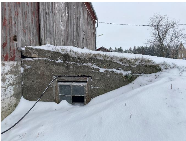
Plate 57: Barn No. 2 wingwall window.
