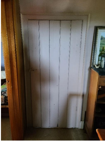
Plate 41: Original wood plank closet door
