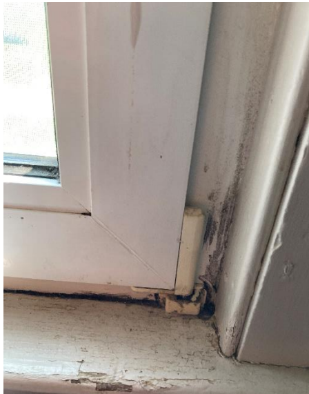
Plate 43: Second storey window
