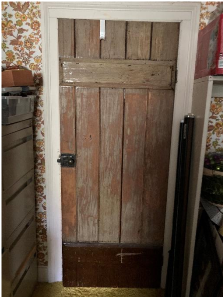
Plate 39: Original wood plank bedroom door
