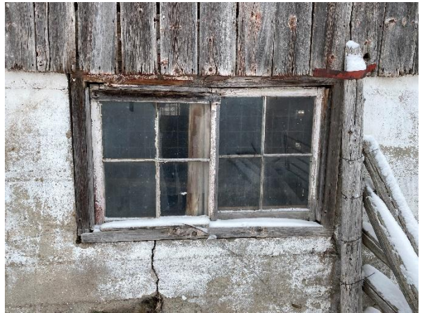
Plate 56: Barn No. 2 window detail.
