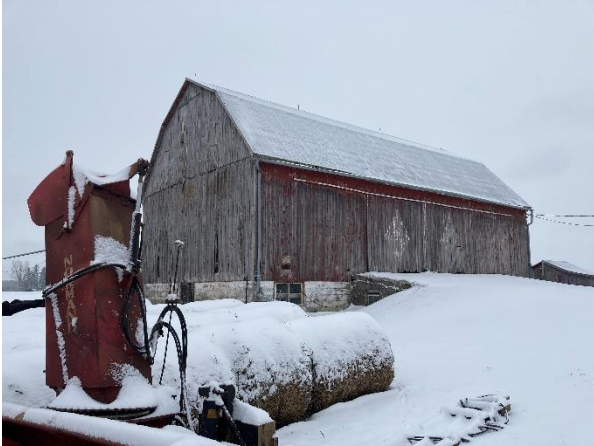
Plate 53: North and west elevation of Barn No. 2.
