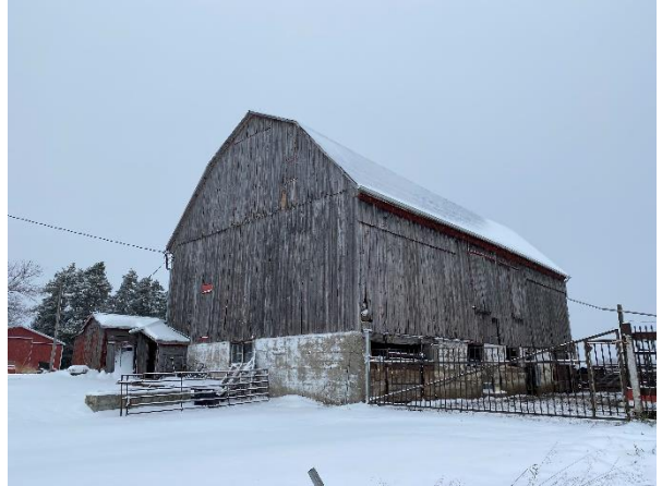
Plate 54: South and east elevations of Barn No. 2.
