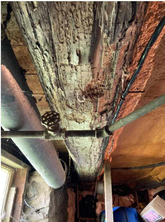
Plate 25: Hand hewn timber floor joist
