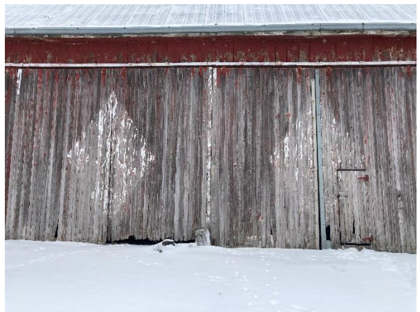
Plate 58: Painted diamond pattern on east elevation ramp doors of Barn No. 2.
